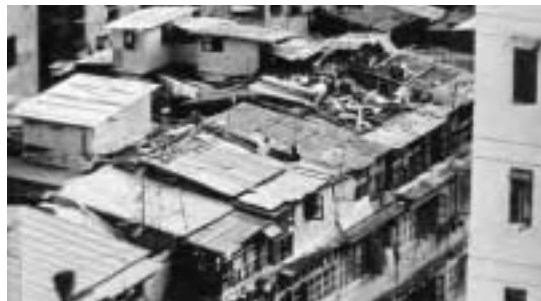
Roof-top squatters in Hong Kong, 1978.
