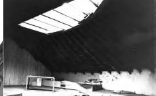
Opening up the roof
